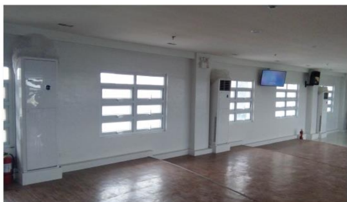
Furnishing of Audio Visual Room of Academic Building (Center Wing)
