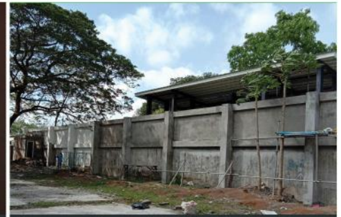
Renovation of Lucinda Campus West Side Perimeter Fence
