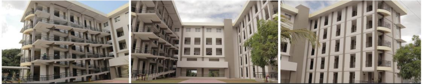
Construction of Academic Building (Right Wing)
