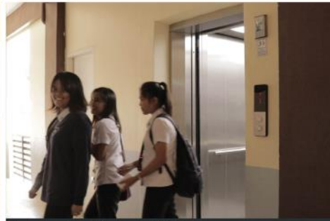
Installation of Passenger Elevator at the CCS Building
