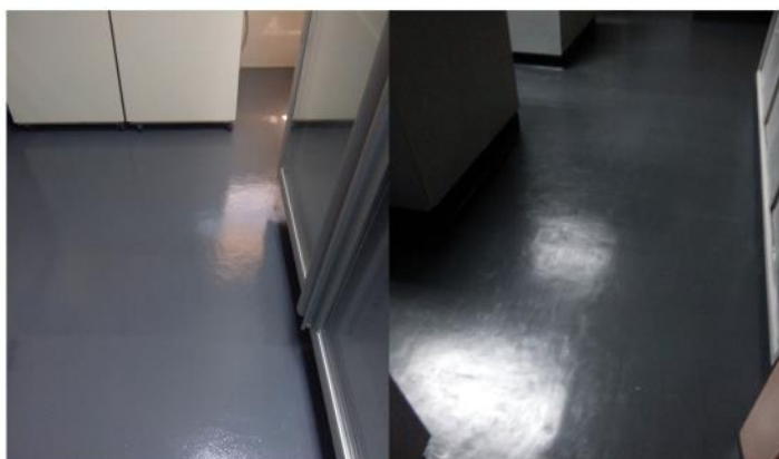
Repair of RED Bldg. Chemical Laboratory Flooring
